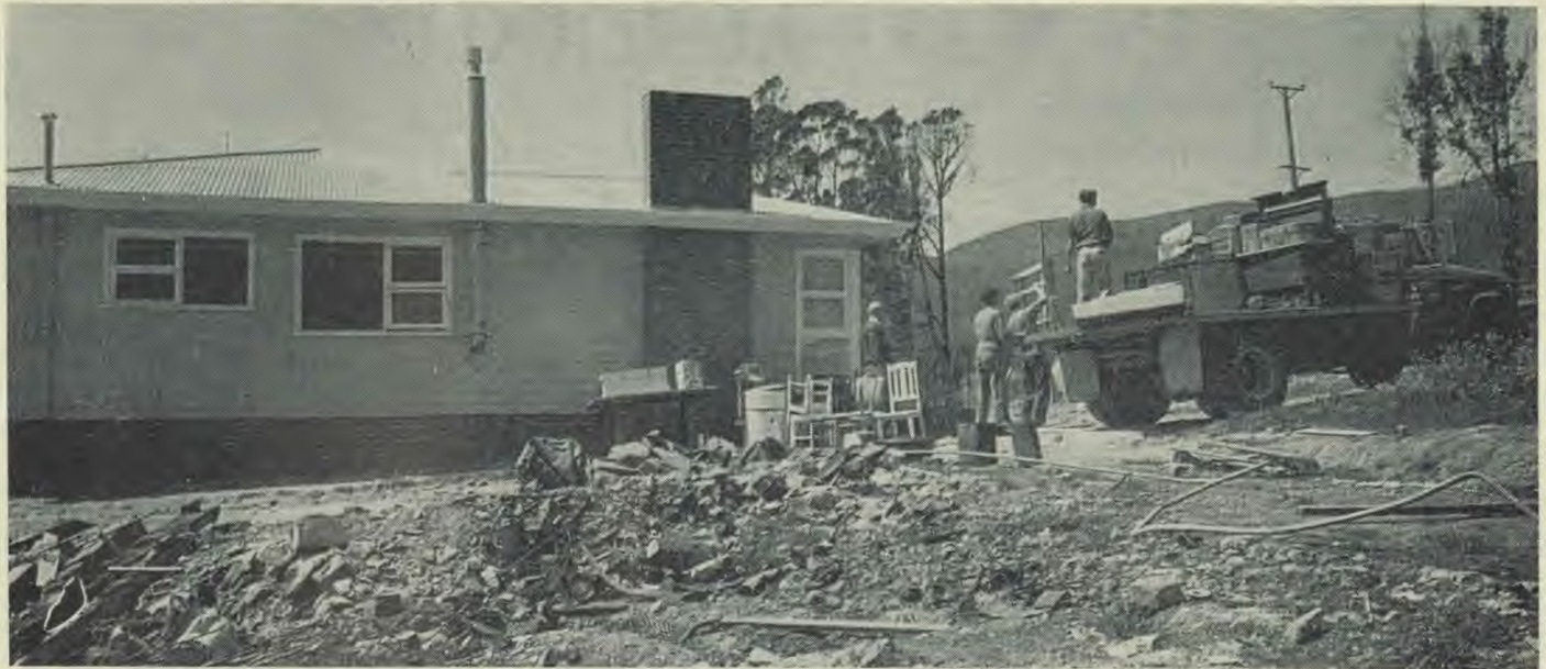
Their new home now stands on the ashes of the old one. Because of the generous help received, a larger home, capable of housing her own family and her parents was able to be built by Mrs. Ivy Zanotti.
