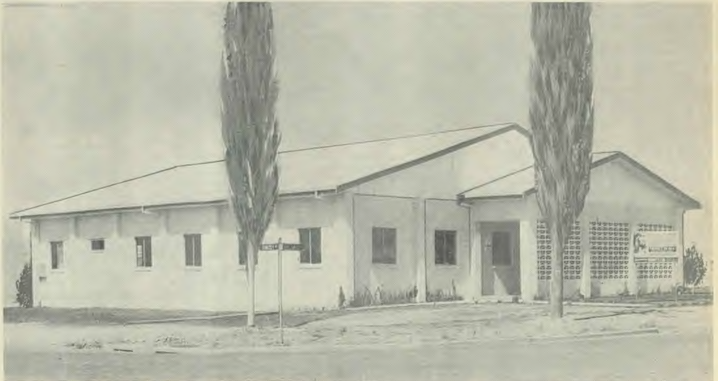
The new Mount Isa church. Our artist has donated the two trees in the picture. Actually they are electric light poles. We thought trees looked better.
