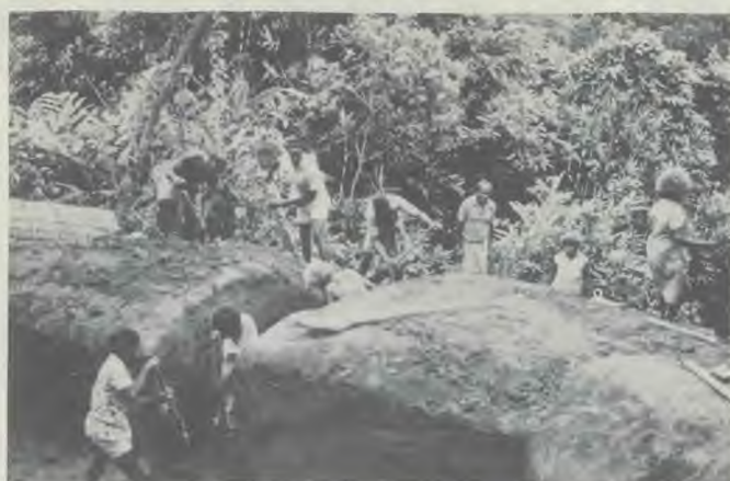
Extensive excavation was necessary to install a new 10,000-gallon fibreglass surge-tank. Photos: D. P. Cobbin.
