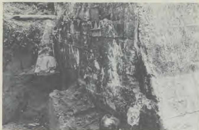
A close-up view of the old, cracked tank which caused so much havoc to the hydro-electric power supply at Atoifi.
