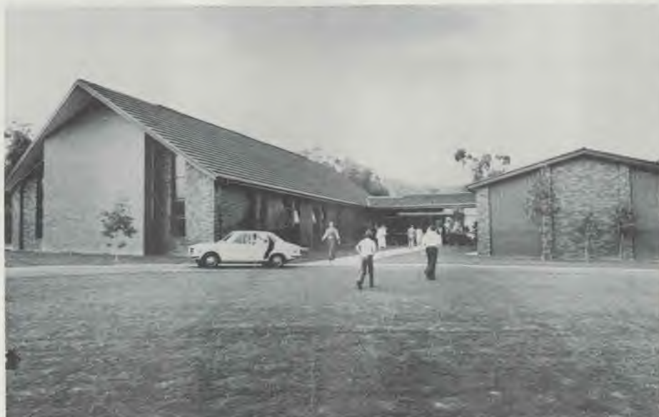
A front view of the recently opened Lilydale church complex. Photos: R. Bowers.
