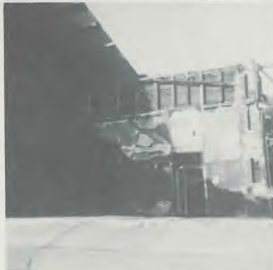
The demolished school. Photos: L. Meaney.
