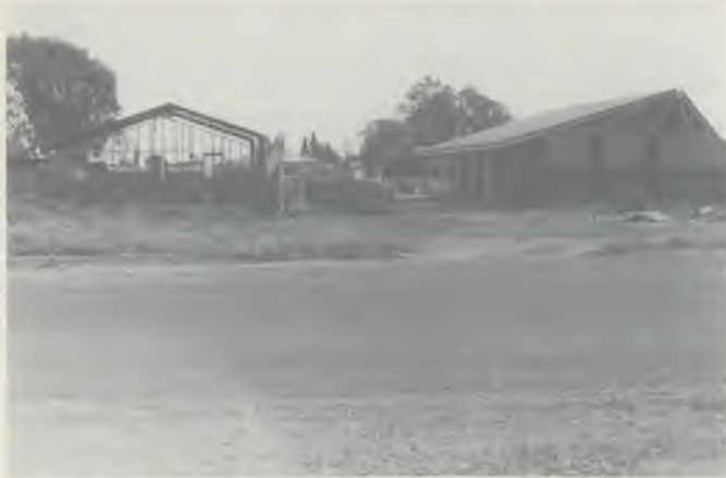
The church and hall complex under construction at Bourke.
