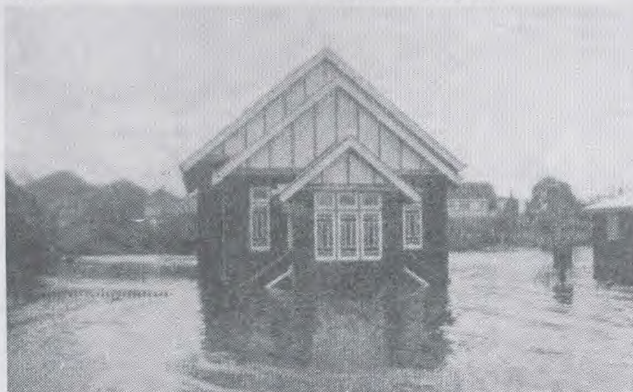
The Bundaberg Adventist church under flood in 1942, less than 12 months after being opened.
