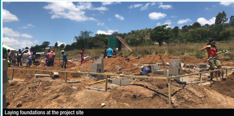
Laying foundations at the project site
