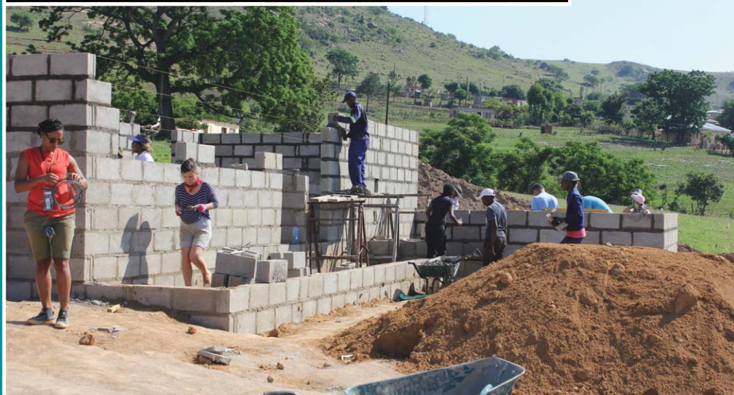
Pre-school halfway through its build
