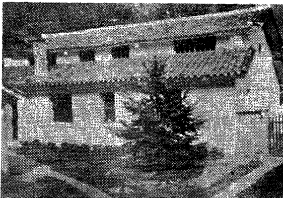
Hospital - Dispensary Building, Tatsienlu. A second floor addition has been completed, giving a suitable operating room and women's quarters.
