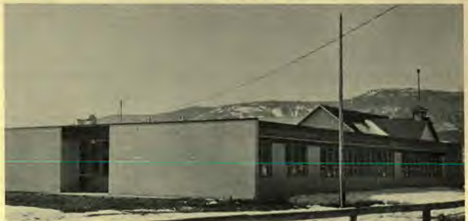
The new North Okanagan Seventh-day Adventist church school building measures 60 x 90 feet and contains four large classrooms, besides other office and service rooms. It is a consolidated school for the Grandview and Vernon Churches.
