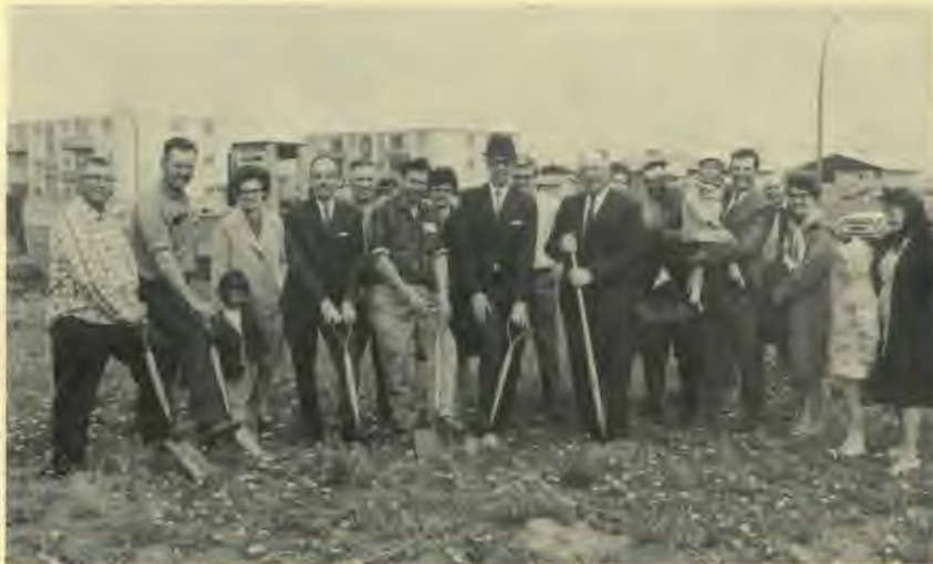
From left to right: Mr. R. Sereda, Ivan Chernipeski, A. Lennox, Geno Astofe, contractor, Ed Chernipeski, His Worship W. E. Fichtner. Some of the membership is seen in the background, as well as those in attendance at the groundbreaking.
