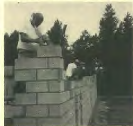
Men work industriously to put up walls.
