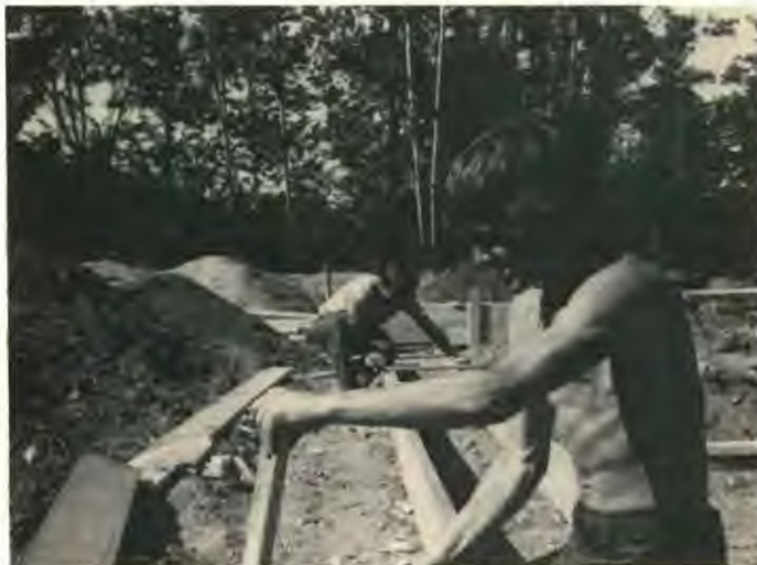
Students Ken Scott and Ronnie Kuppers help layout of footing forms.
