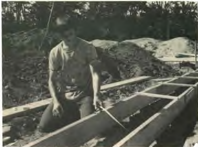
Ronnie Kuppers, grade 10, places forms for footings.
