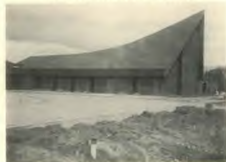
New Kelowna Church under construction.
