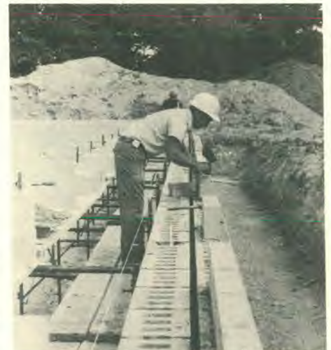
Workmen laying block for the Kingsway Pioneer Home in Oshawa.
