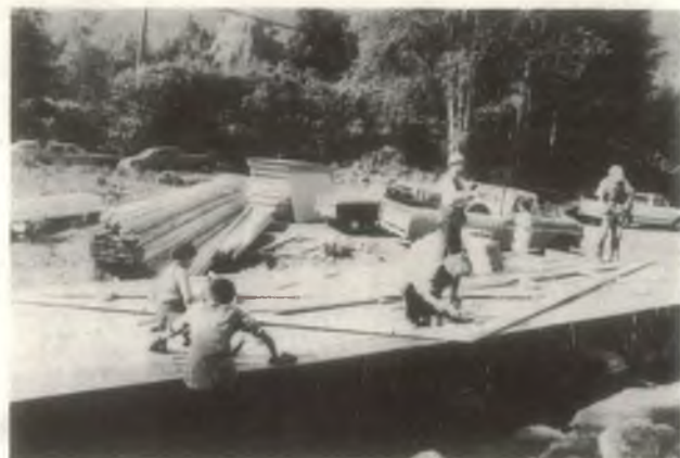
Crew assembling one of the 64 trusses, of which approximately 50 were made in 1 day.
