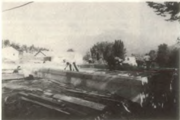
Laying out the main walls on the 1st day — all 4 walls. Several interior partitions were up at the end of the 1st day of the B.C.'s Chapter 1st Maranatha Flights project.
