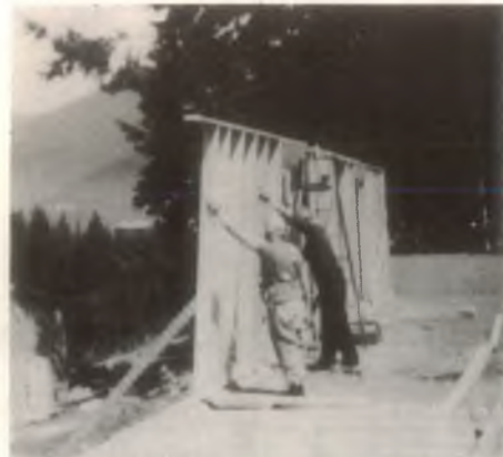
1st wall being erected by local members.
