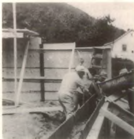
Total concrete helps put the church on a solid foundation. Brothers Sorenson, Jay, Pond and Edey direct concrete into the foundation.
