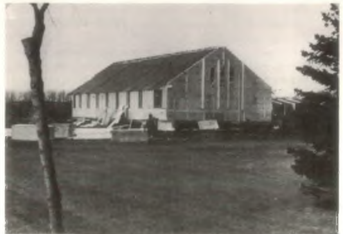
Re-assembled and approaching completion.
