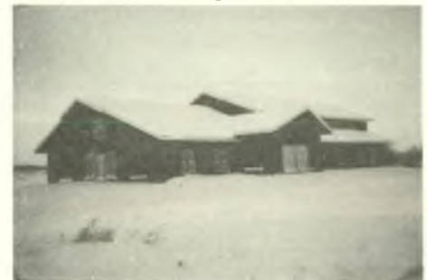
New church building accommodating the Peoria and Smoky church members.
