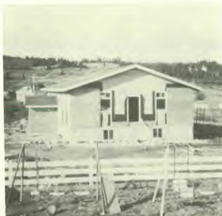
New church school under construction at Bay Roberts, Nfld.
