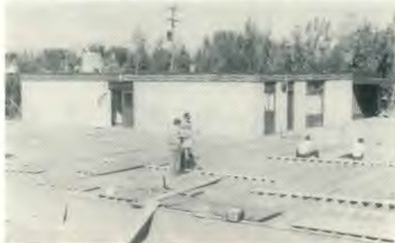
The work done by volunteers will save thousands of dollars in labour costs. Here the sub-floor is being laid.
