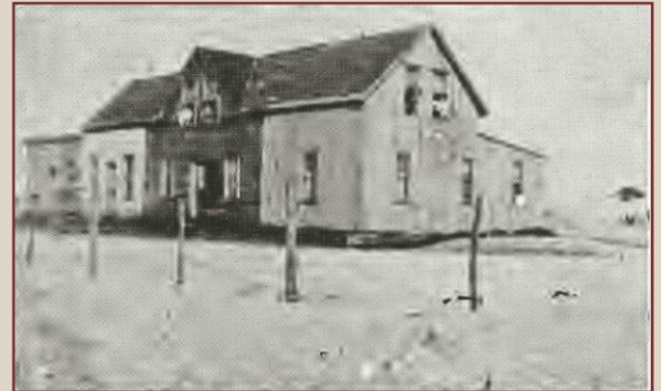
The school building on the farm in Leduc, Alta. Canadian Union Messenger , Vol. 41, No. 17, p. 4
