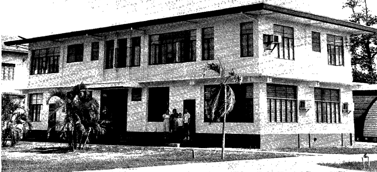
The new North Philippine Union guest house, located in Pasay City. In addition to guest apartments and guest rooms, there is also a schoolroom for the children of the overseas families.
