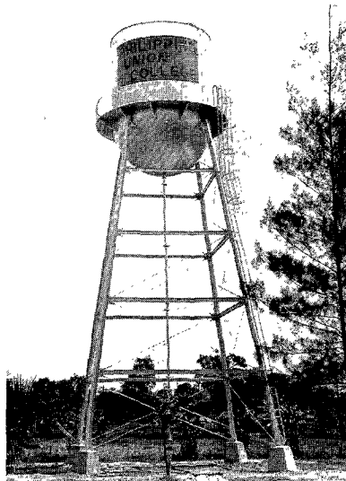
The new water tank on the campus of Philippine Union College. The tank holds 30,000 gallons of water.
