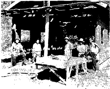
Ministers, church officers and laymen joined hands in building the chapel in barrio Cabacungan, La Castellana, Negros Mission. Money and labor were donated by brethren and friends.
