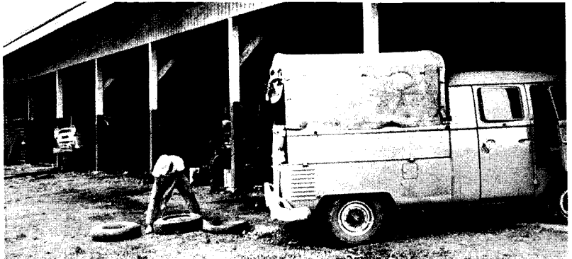
CARS. This is the newly-constructed garage at Mountain View College in the Philippines.
