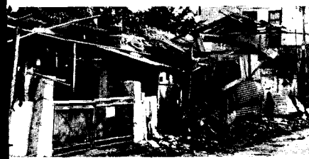
ALLEY. Dwellings along an alley between the mission compound and the Saigon Adventist Hospital looked like this after the battle.
