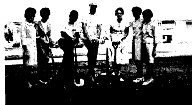
BUILDING. Work is in progress on the Ps. 75,000-annex to the office building of the North Philippine Union in Pasay City. Breaking the ground with Pastor T. C. Murdoch, Union president, are, left to Thelma Kintanar, office secretary; M. G. Jereos, Union Secretary and Amy Sherrard, Assistant Educational secretary for Parent and Home, as three other office secretaries look on.
