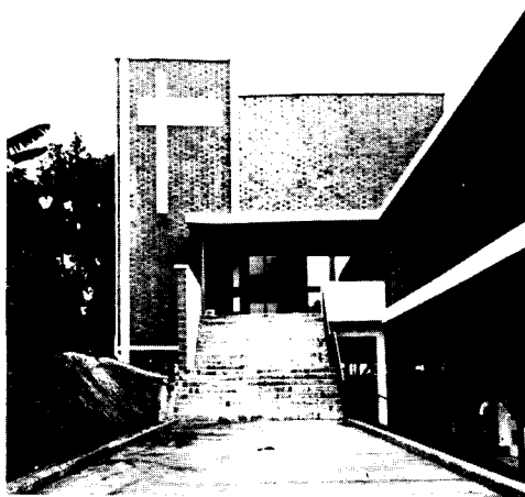
Front entrance to the Auditorium. The balcony on the right flanks the old chapel, now being converted into a college building for classrooms and administrative offices.
