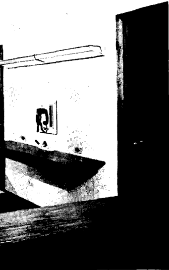
veniently located on the new wing.
