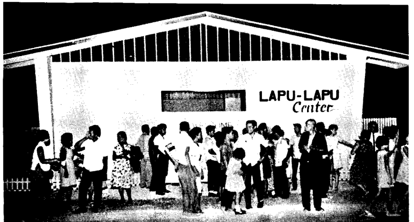
CENTER. This is the front view of the Lapu-Lapu Center where evangelistic meetings were conducted by Pastor D. M. Niere.
