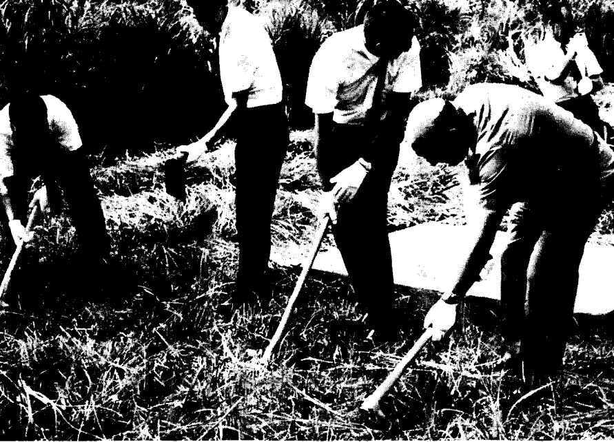
GROUP. The ground is finally broken for the new Servicemen's Center on Okinawa.
