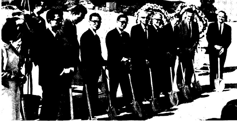
SOD. Pastor Wendell Wilcox, center, Chairman of the Board of the Seoul Sanitarium and Hospital, and other hospital officials break ground for the new million-dollar hospital building project.
