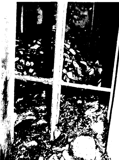
DESTRUCTION. Approximately US $12,000 worth of property was destroyed during the fire which gutted two rooms of the Korean Publishing House.
