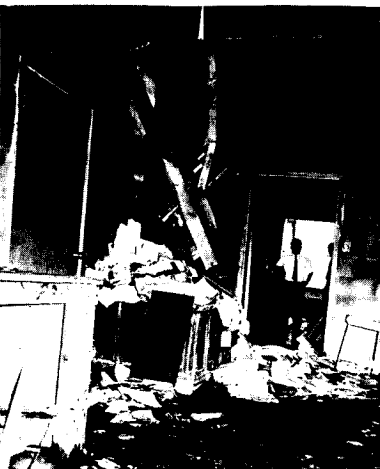
REMAINS. The fire left its mark with fire and smoke stains and the water by the firemen.
