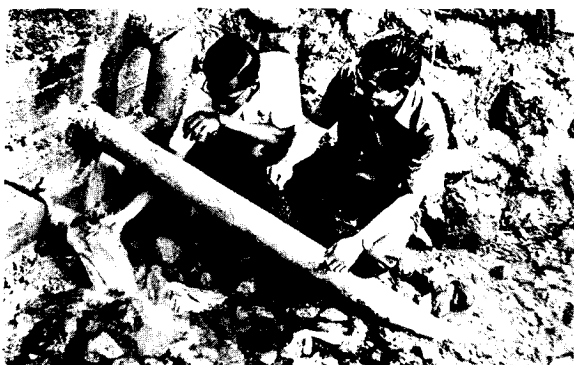
WATER! Four-inch pipes 1,521 meters long connect the Naga View Campus of Philippine Union College with a spring 378 feet high. The water reached the campus September 13, their big "water festival" day. Feeling the gush of the water is Oscar Palomero, school engineer, while Associate Dean J. B. Villagomez looks on.
