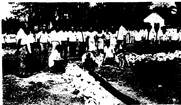
FIRST STONE. The mission staff and school faculty watch as the mission president lays the first stone for a new classroom-laboratory building at North Sumatra Academy.
