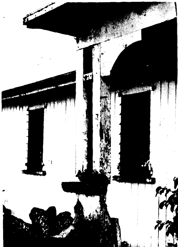
Decay has taken over this section of the boys dormitory at Fulton College. Existing dormitories were originally built during World War II from used materials.
