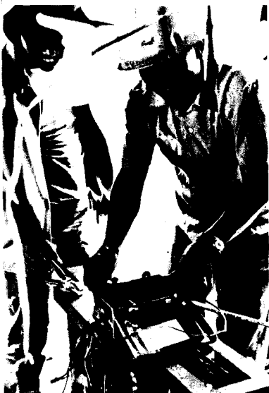
Porteza shows a student how to connect temporary electricity for the power plant. The new plant will put out approximately 450 kilowatts at the lowest output whereas the present plant gives a maximum of 150 kilowatts. Among other things, with the new electric plant, the college hopes to expand the broadcast hours of radio station DXCR.
