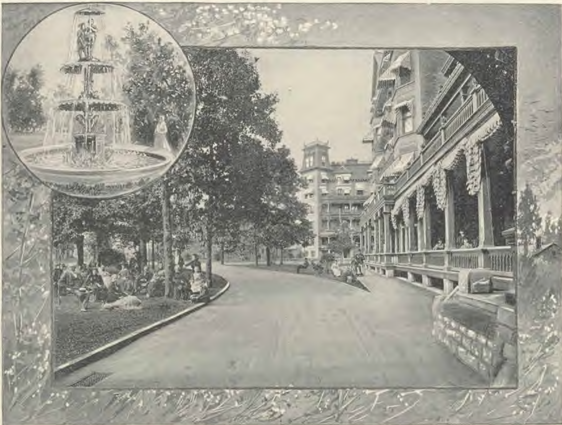
View of the Front Drive, Looking North from Main Entrance.
