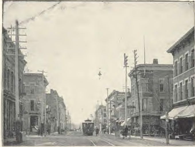
JEFFERSON ST., LOOKING SOUTH.
