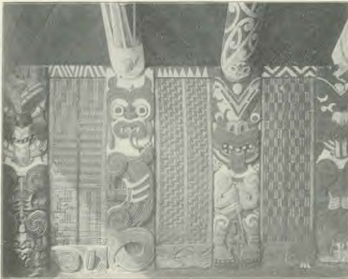
SIDE WALL OF A MAORI SCHOOLHOUSE, COMPOSED OF CARVED UPRIGHT PILLARS CONNECTED BY WOVEN MATTING.
