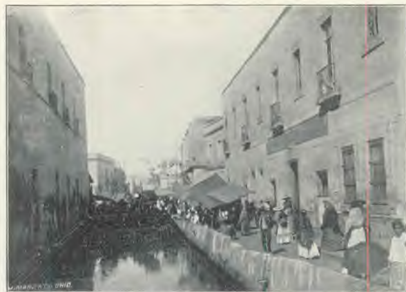
LA VIGA CANAL, NEAR CITY MARKET.
