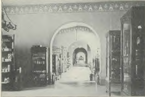
FOODS AND FILTER ROOM.
