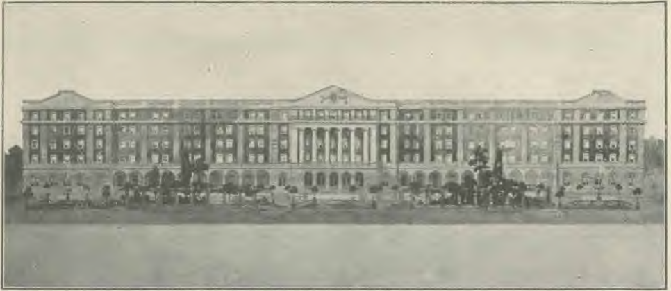
The New Sanitarium, to be Completed in May, 1903. 560 Feet Long. Accommodations for 1000 Guests.
