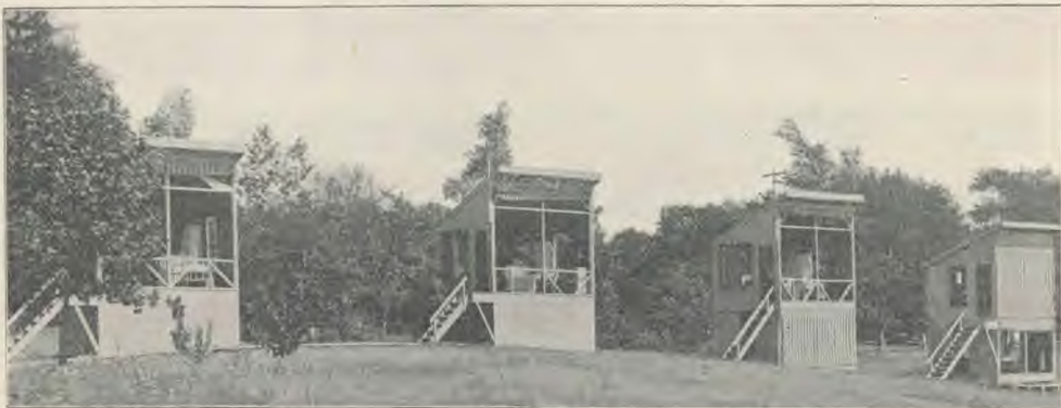
INDIVIDUAL SLEEPING SHACKS USED IN A MASSACHUSETTS SANATORIUM
