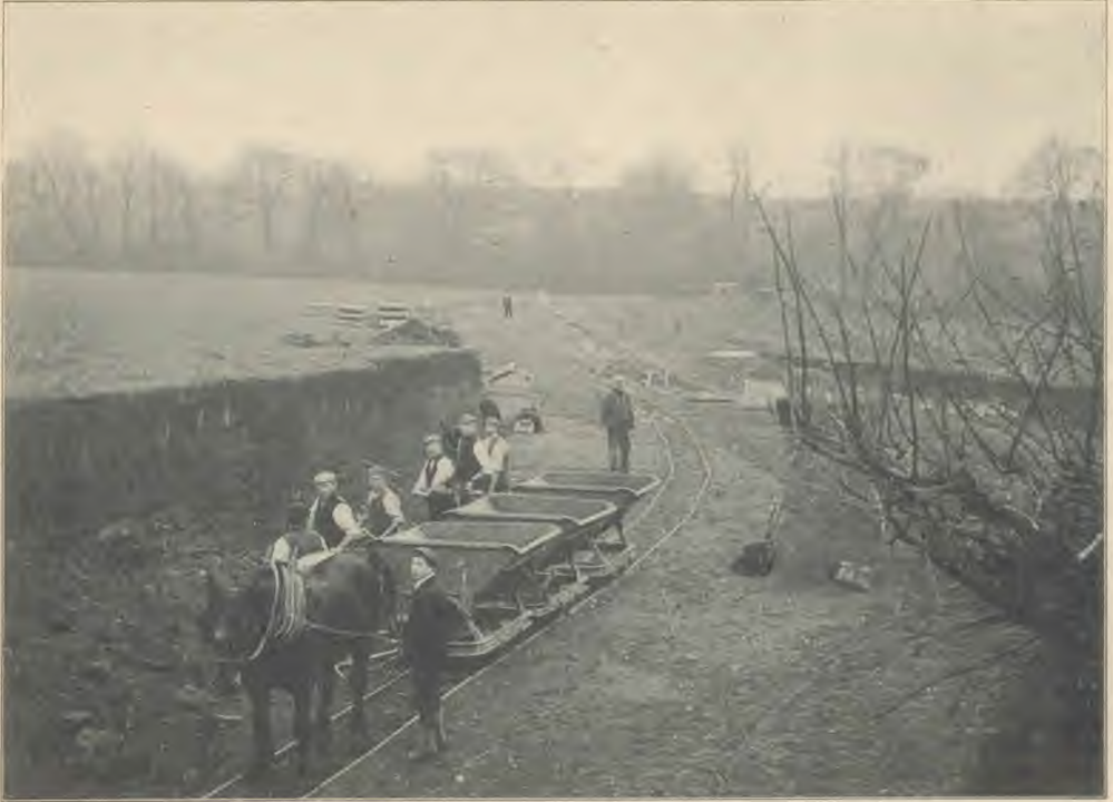
LAYING OUT NEW ROADS IN THE GARDEN CITY
