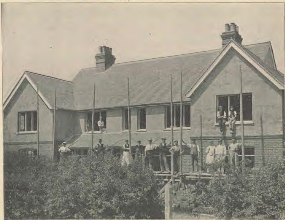
COTTAGES IN COURSE OF CONSTRUCTION
