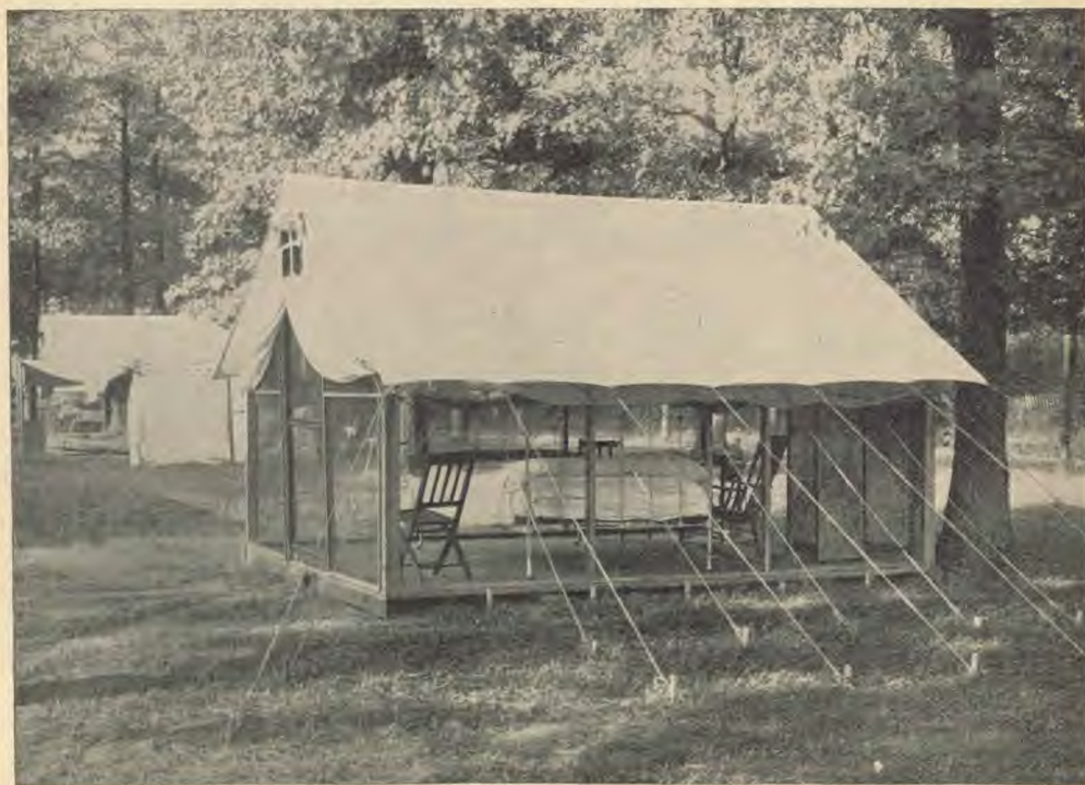
A Bedroom Tent in the Back-yard with Wire Screen Frame (A Connection with the House Lighting System Made Possible the Lighting of the Tent by Electricity)
