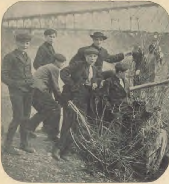
Under the Viaduct
