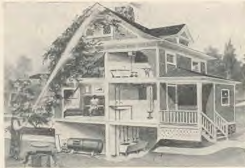
Kewanee Water Supply Outfit in Operation
