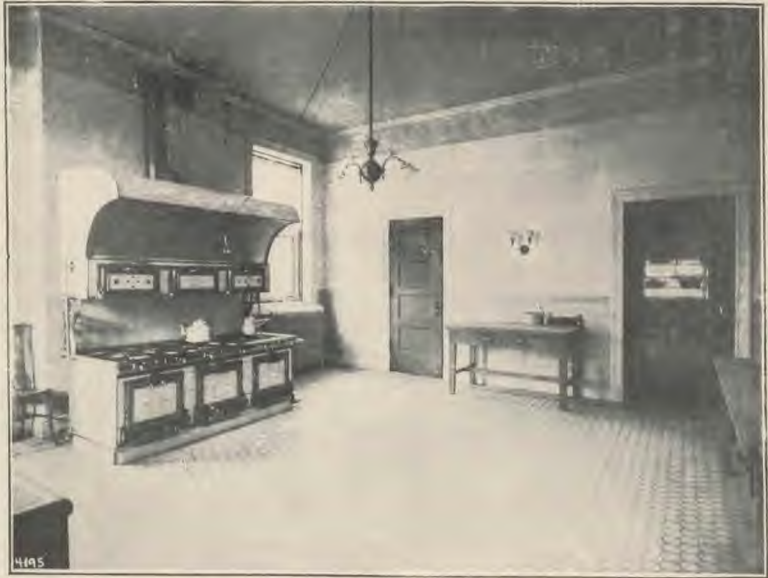
A Kitchen Floor Completely Tiled
