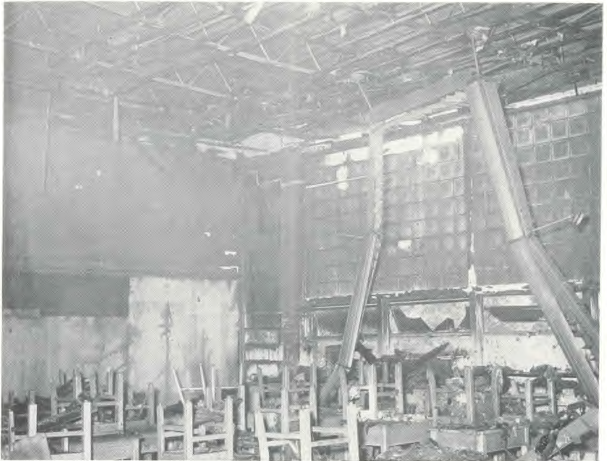
One of the classrooms. Note the lack of burning of the contents. Can you visualize the difficulty in trying to escape via this type of window?
