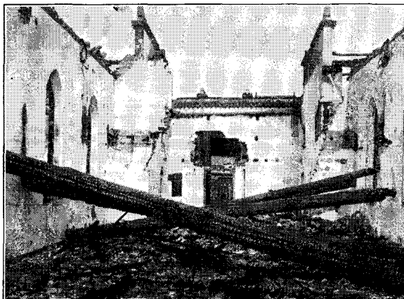
THE NORWEGIAN CHAPEL IN CHANGSHA COMPLETELY DEMOLISHED BY THE RIOTERS OF 1910.
