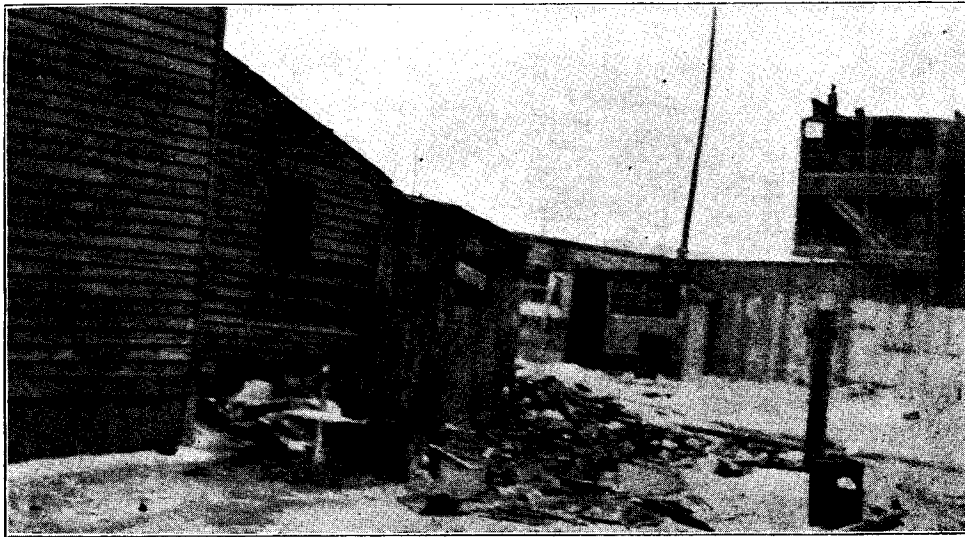
Rear View of house in which a family lived until house was condemned recently because of unsanitary conditions.
