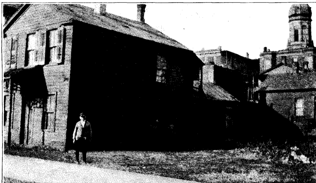
A Dilapidated Dwelling House in the Hinsdale Nurses' Center District.
