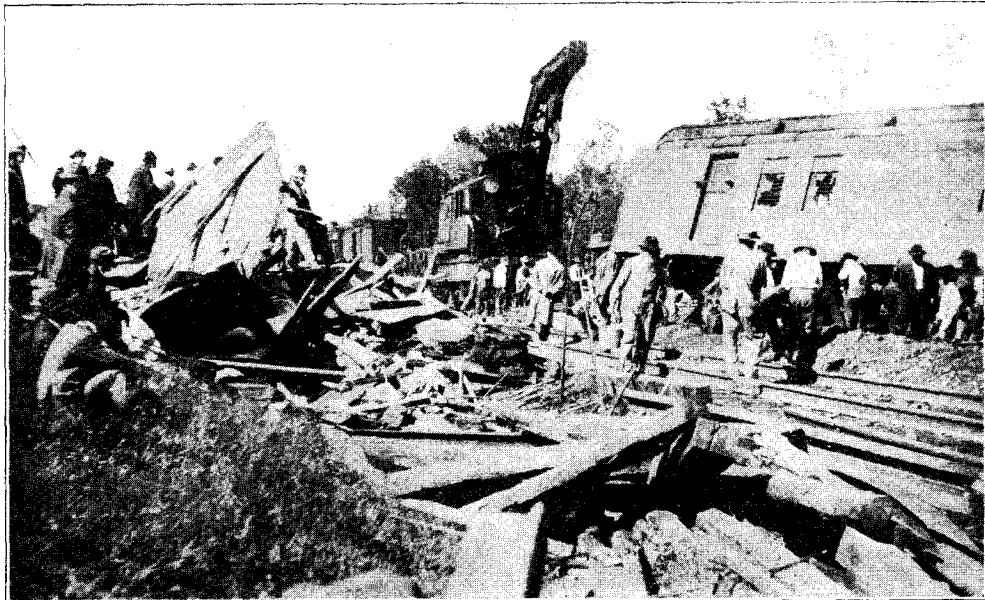
CLEARING UP THE WRECKAGE
