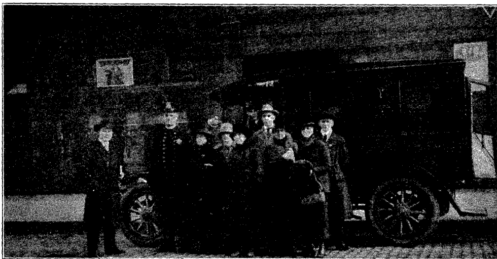
View of Our Jail Workers, Taken in Front of the Clark Street Station
