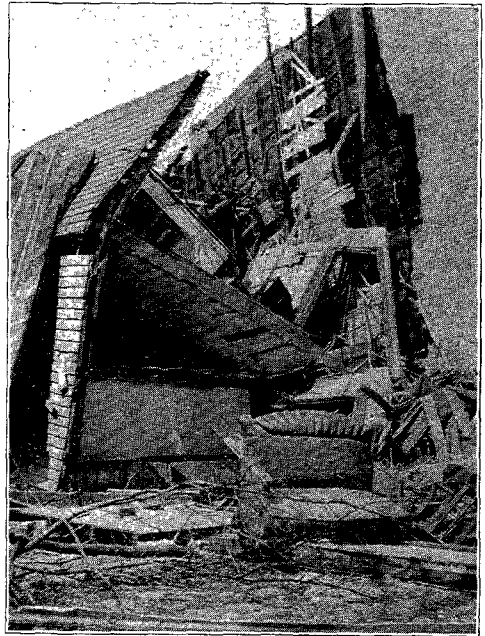
Wreckage Caused by the Recent Tornado. View Taken Only Twelve Miles from Hinsdale.
