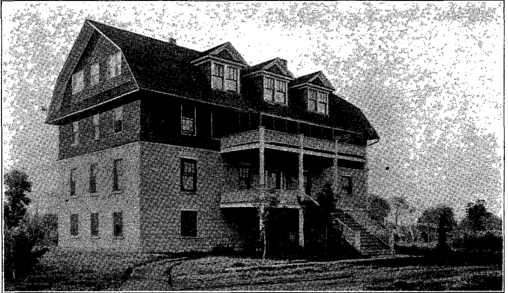
The Building, Now Being Remodeled for the Home Family.
